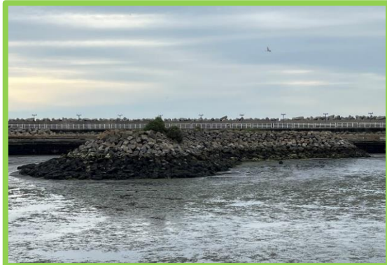
Rock revetment breakwater in good condition bar mature vegetation growth (/C0401C30)
