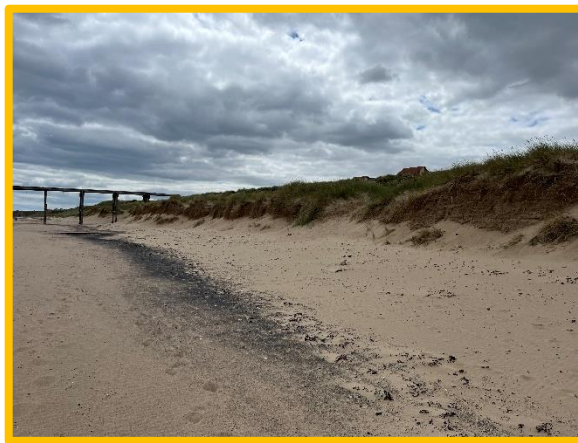
Dunes locally poor adjacent to Steetly Pier (/C0302C01)
