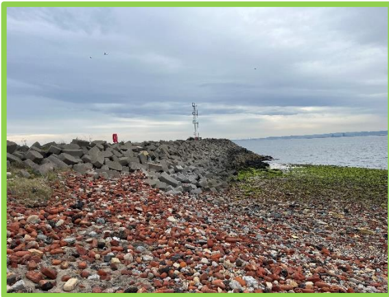
Middleton Jetty south aspect. Buildup of construction rubble in the foreground (/C0401C16)
