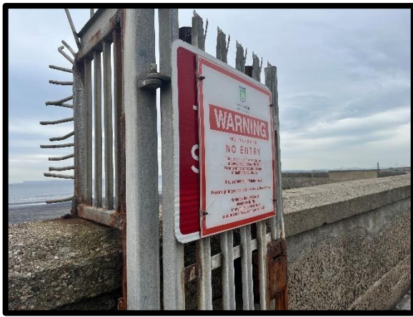
North Pier signage (/C0401C22)
