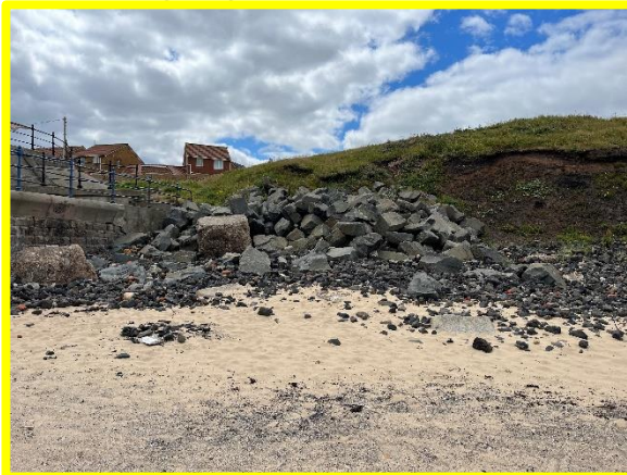
Rock armour revetment at Marine Drive seawall (/C0302C03)
