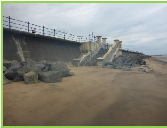
Northern access steps (/C0501C05)
