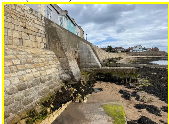
Recently constructed outfall and abutment. (/C0401C35)
