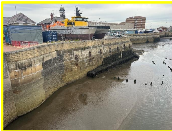
Local repairs to masonry seawall to north of harbour entrance (/C0401C24)
