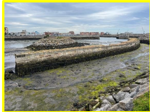
Old quay wall structure in fair condition (/C0401C31)
