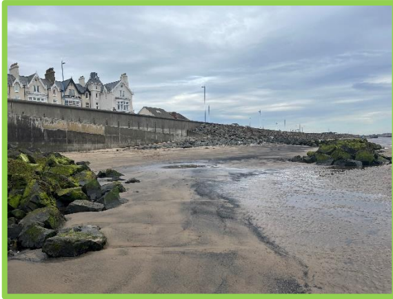
Exposed rock armour berm at Little Scar access ramp (/C0401C33)
