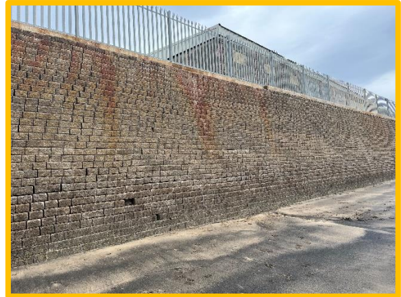
additional block loss (/C0401C19)
