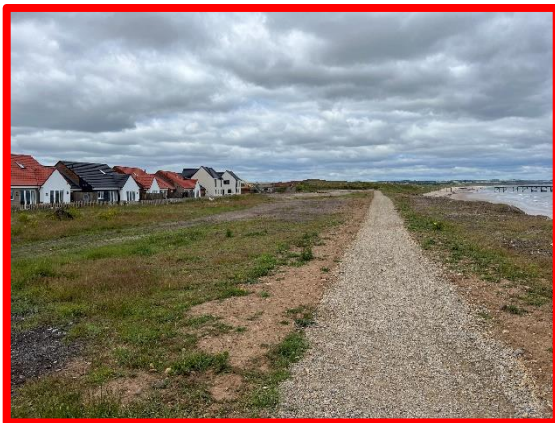
Property development on former industrial site, fronted by collapsed gabion structure (/C0302C02)
