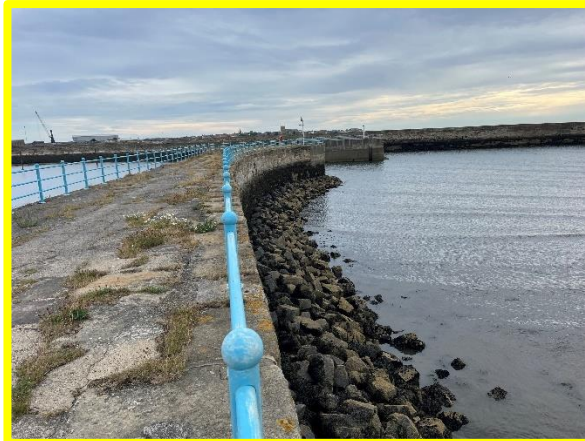
Rock armour against outer face of Middle Pier (/C0401C28)
