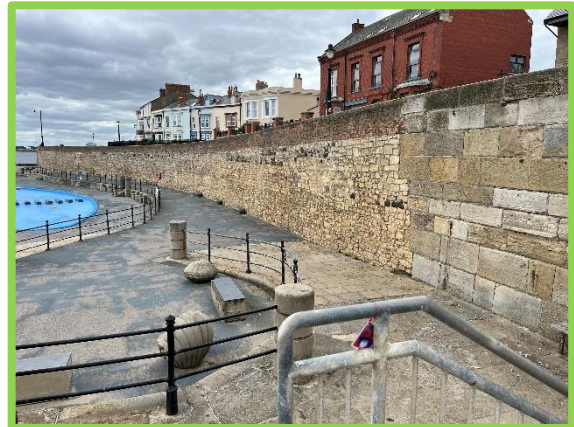
Rear masonry wall in fair to good condition (/C0401C03)
