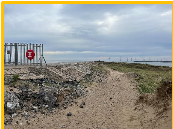
Southern aspect of North Gare Breakwater (/C0503C01)
