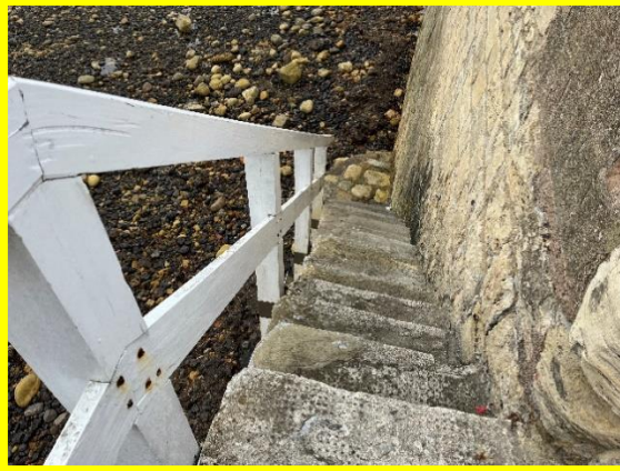
Repaired handrailing and beach access steps (/C0401C35)
