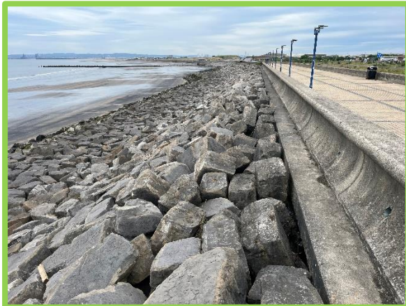
Rock armour revetment and concrete seawall (/C0401C33)
