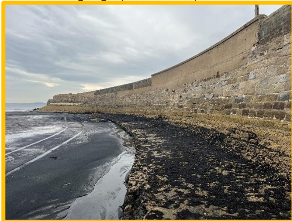
North face of North Pier (/C0401C22)
