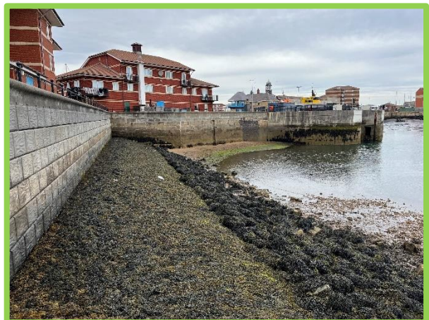
Concrete blockwork revetment obscured by vegetation (/C0401C25)
