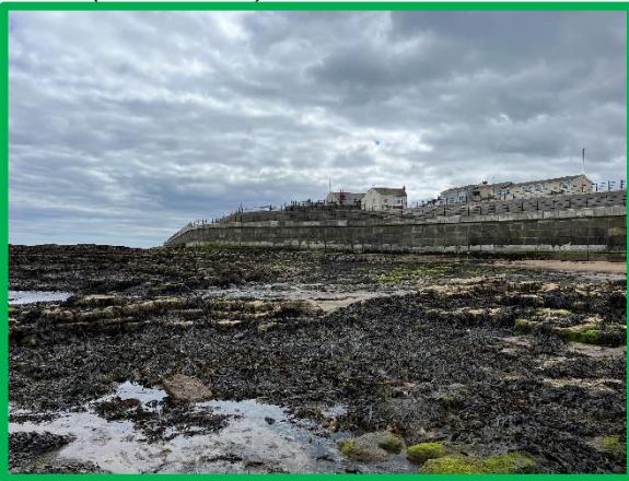
As built condition sea wall – inaccessible foreshore to the south. (/C0303C02)
