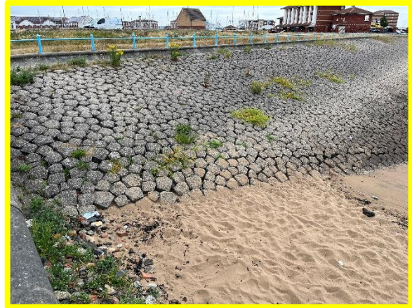
Steeper profile to the south (/C0401C26)
