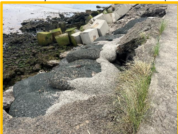
Concrete blocks and bagwork repairs to voiding.(/C0503C01)
