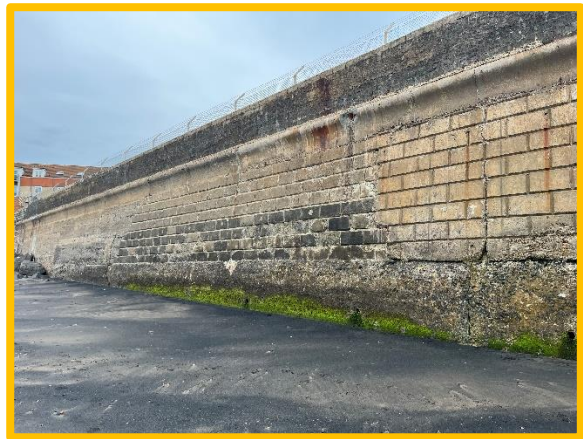
Vertical crack through parapet and seawall (/C0401C20)
