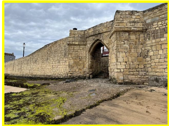
Town Wall benefiting from recent repointing works (/C0401C35)
