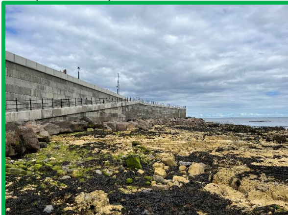
As built condition seawall (/C0303C04)
