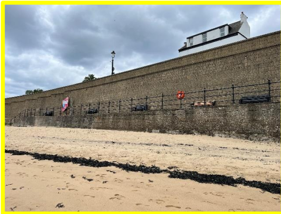
Town Wall benefiting from recent repointing works (/C0401C35)
